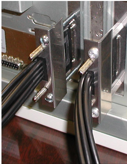
Figure 2-1: Installed Cards with Stability Bracket Accessories
